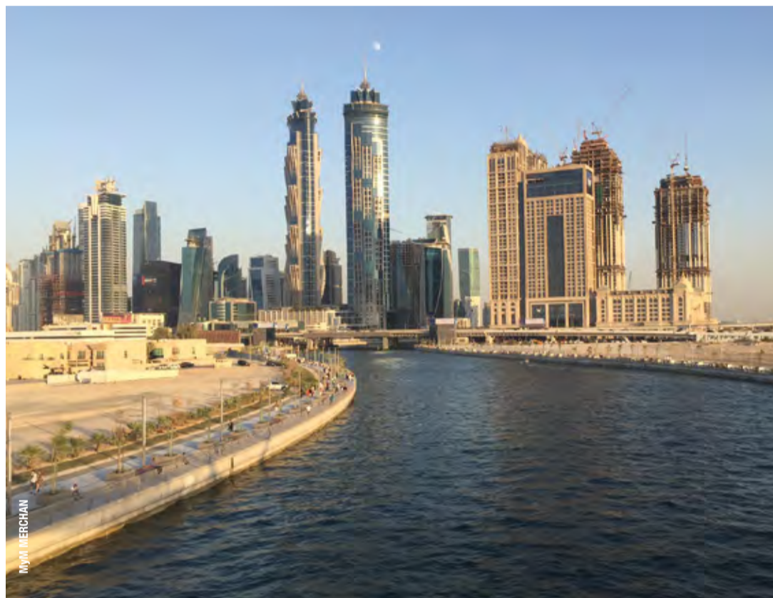
The construction of the Dubai Water Canal that turns the city centre into an island took two years and 516 million euros. Opened in November 2016, it has become a new attraction for tourists and residents alike.
