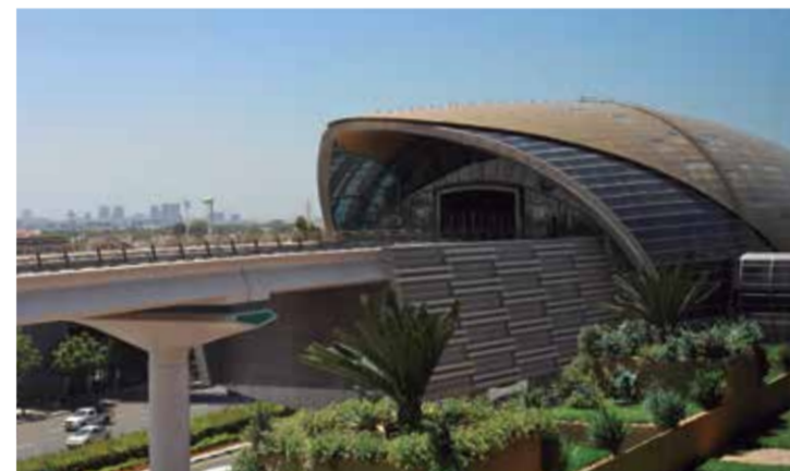
Image of Dubai Metro, owned by the Roads and Transport Authority (RTA) of Dubai. Photos: MyMMerchan.
